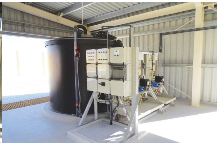
FeCl3 Dosing Unit (side view)
