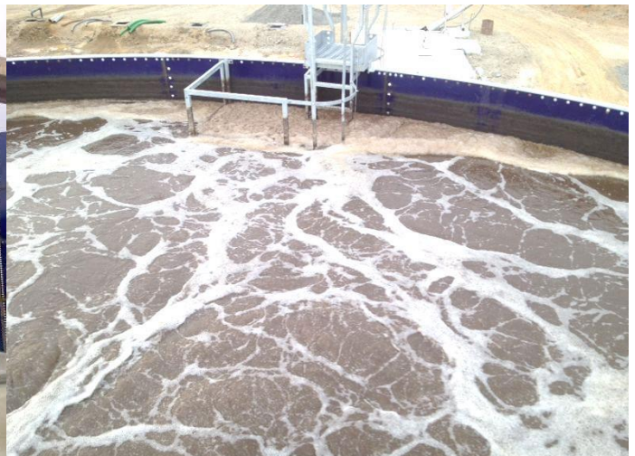
Aerobic Tank
