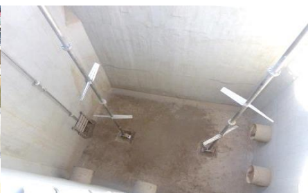
Construction of new main mixing & distribution chamber
