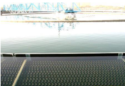
Installation of lamella settlers in 8 clarifiers
