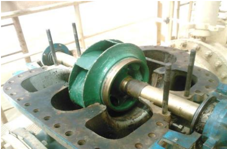
Overhaul of 11 intake pumps and 13 low-lift pumps
