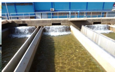
Repair or new construction & automation of 36 sand filters
