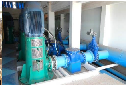
Installation of 6 low-lift pumps including headers
