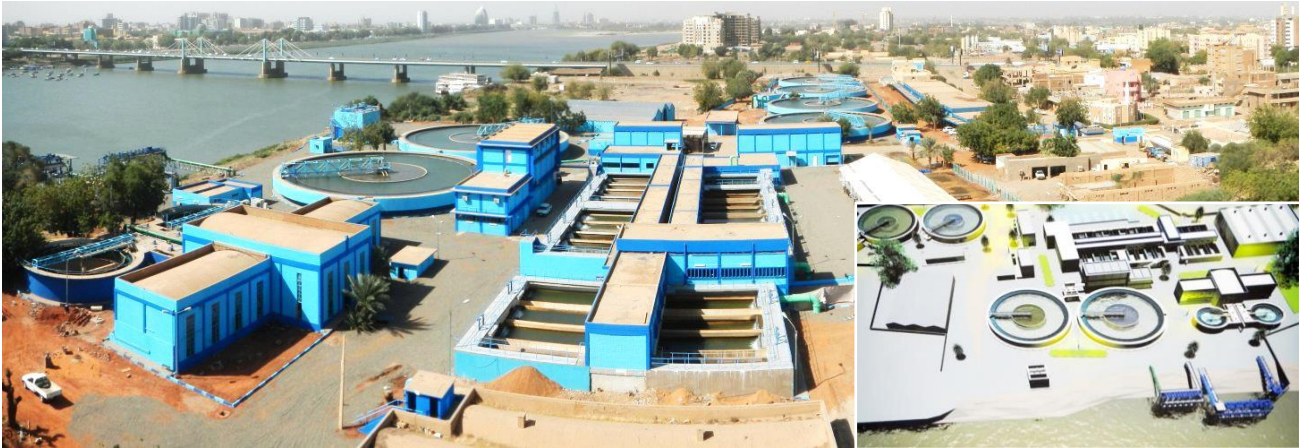
Repair of 8 clarifiers:
