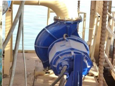
Installation of 8 new river intake pumps & pipelines
