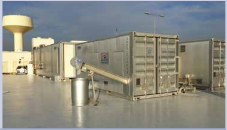
Brackish Water Reverse Osmosis System 300 m 3 /d , Moskau, Russland
