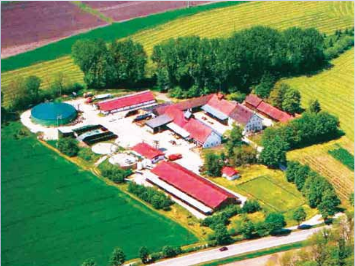
Biogas plant - 700 kW - manure and waste
