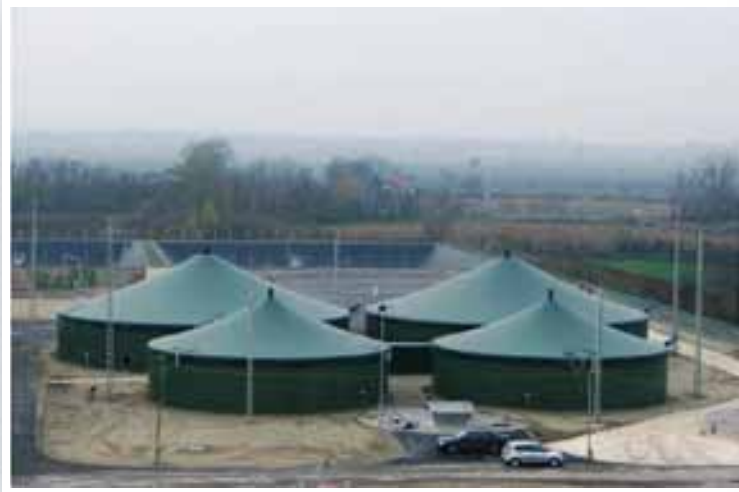
Biogas plant - 1.4 MW - food waste
