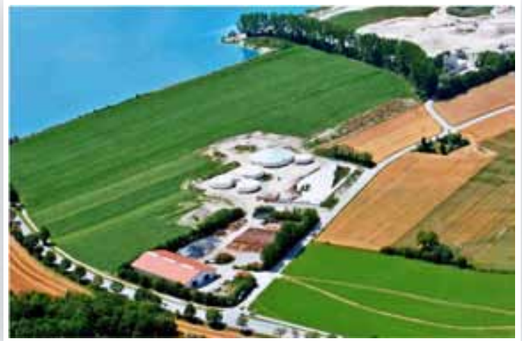
Biogas plant - 500 kW - manure and silage
