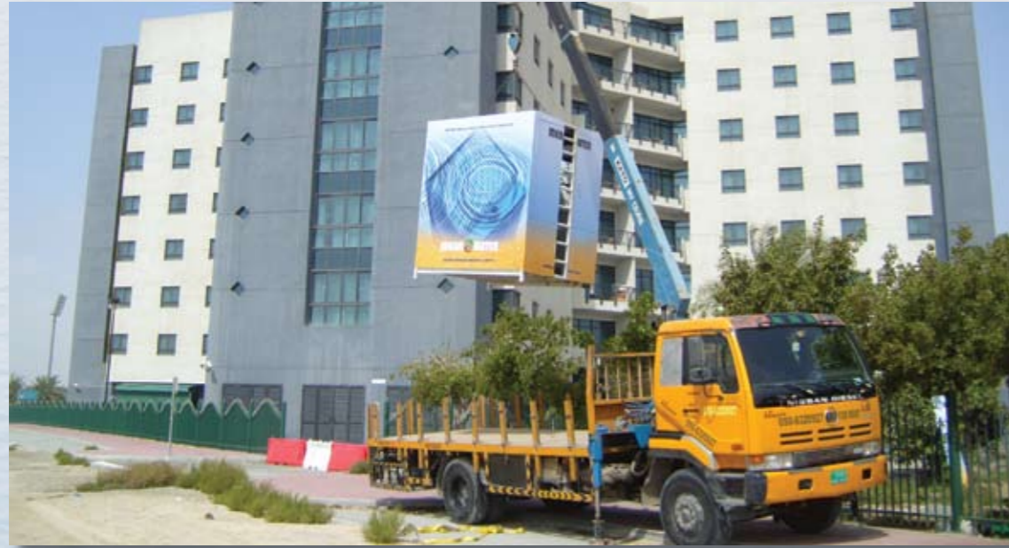
Unloading of MBR Pilot Plant at test location
