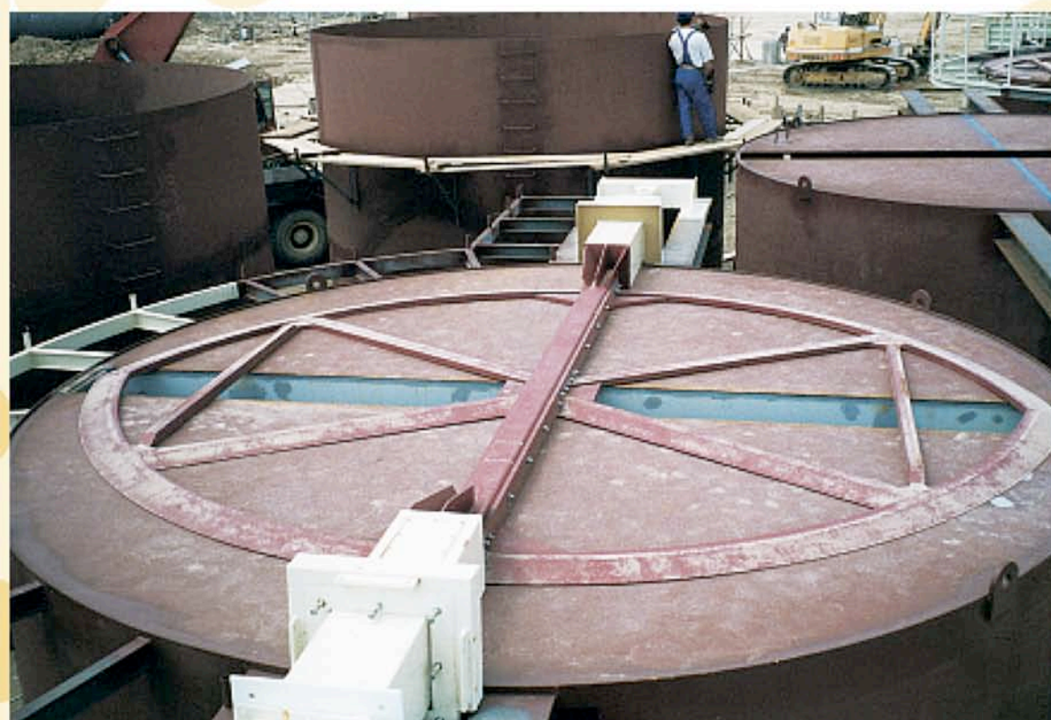
Installation of tandem Sliding Frame for wood material in 6000 mm diameter silo during silo construction.
